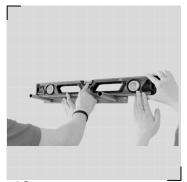
Please ensure the bracket is level using a spirit level. Mark the locations of the holes on the bracket and make sure to secure it to at least one stud.
