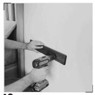
Secure the bracket to the wall using screws appropriate for your wall type.
