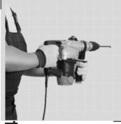
If you are not mounting the bracket to a stud, you will need to use wall anchors. Drill a hole suitable for your wall type and insert the anchor.
