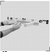
Please ensure the bracket is level using a spirit level. Mark the locations of the holes on the bracket and make sure to secure it to at least one stud.
