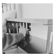
Mark the hole positions on the bracket and ensure it is secured to at least one stud.
