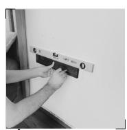
Make sure the bracket is level using a spirit level. Mark the hole positions on the bracket and ensure it is secured to at least one stud.
