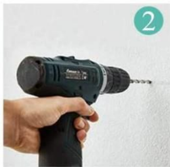
2. Drill a hole at the mark
