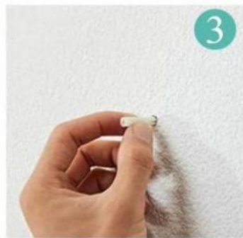
3. Insert expansion tube
